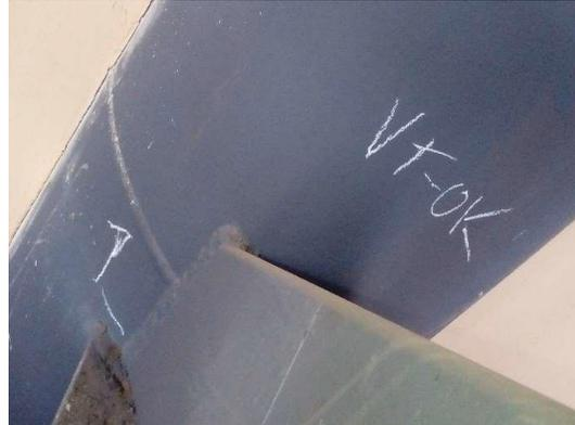
**UNIONES DE VIGA A COLUMNA TUBULAR**
